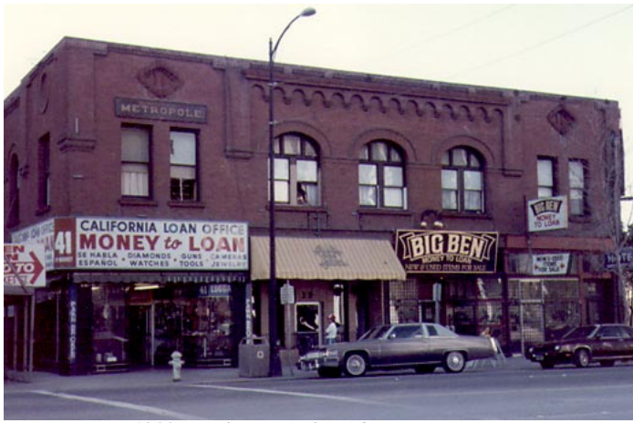
1903 Hotel Metropole undergoing renovation
