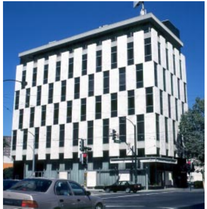
1960s Pestana Building Being Prepared for Demolition Photo by April Halberstadt
