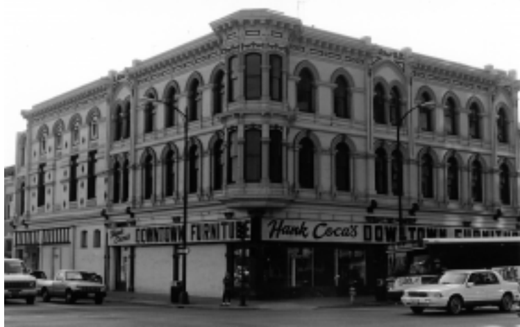
Odd Fellows Building Third and Santa Clara Streets Photo courtesy of Jack Douglas
